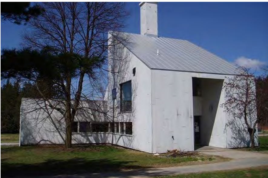
Front and south side of Sawtell House (#22)
