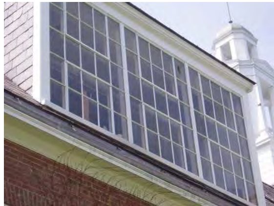
Historic windows: Left photo of eight-over-eight window with wood brick mold, modern storm window. Note grapevine joints in brick masonry. Right photo of original steel window in shed dormer.
