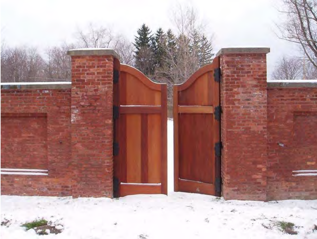
New doors and repointed east wall.
