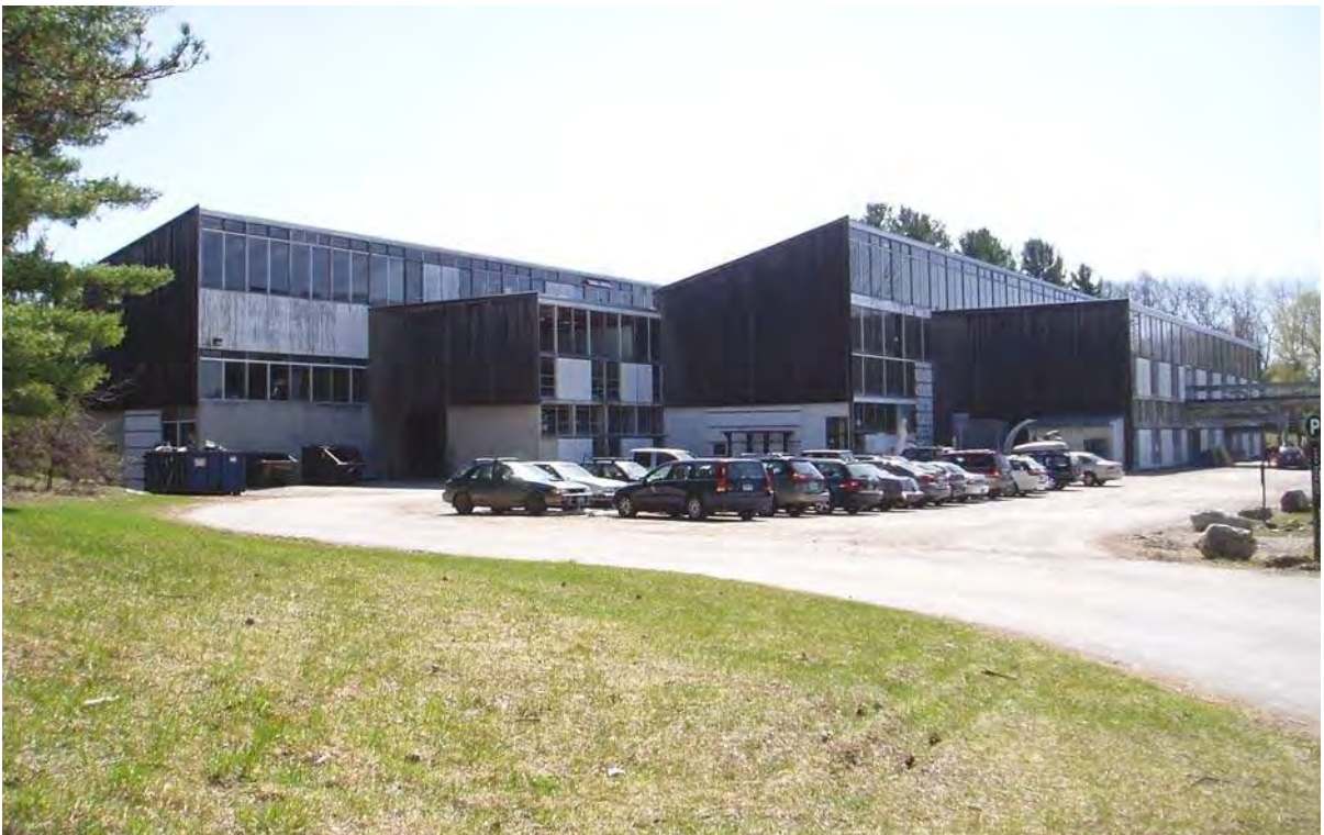
View of rear elevation looking southwest.
