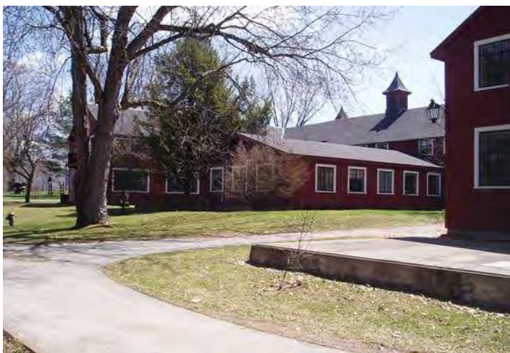
View looking southeast of c. 1939 north extension (left) on east wing, and c. 1970 center extension (center).
