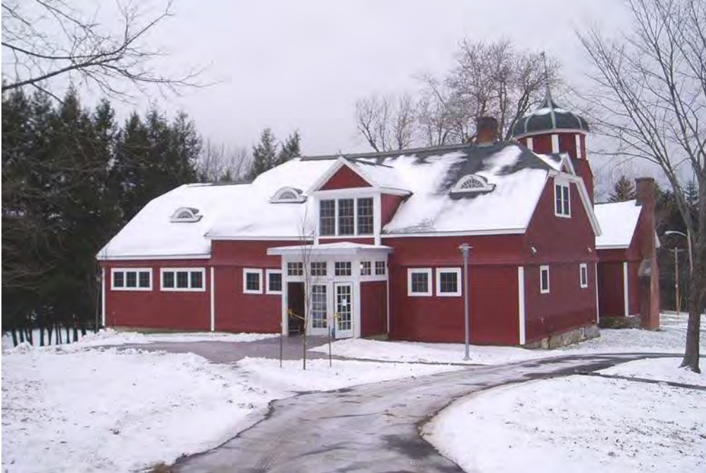
East elevation showing new entry vestibule.
