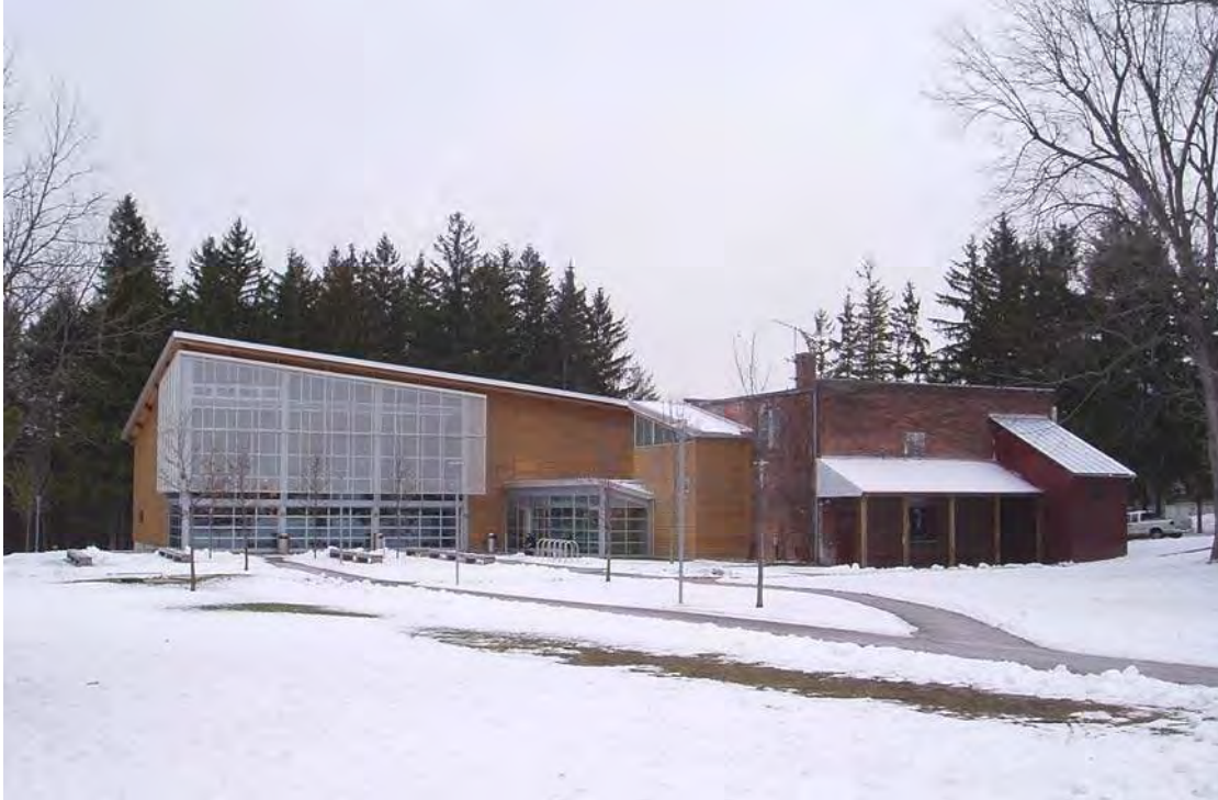
View looking west of new Student Center on left, former brick garage on right.
