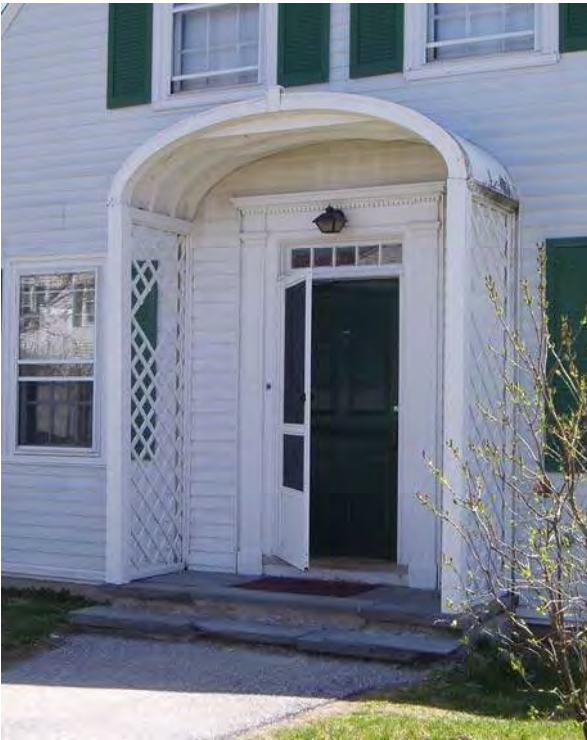
Stokes entry on front gable.
