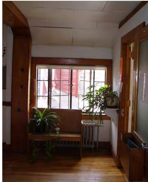
View of east wing, second floor.
