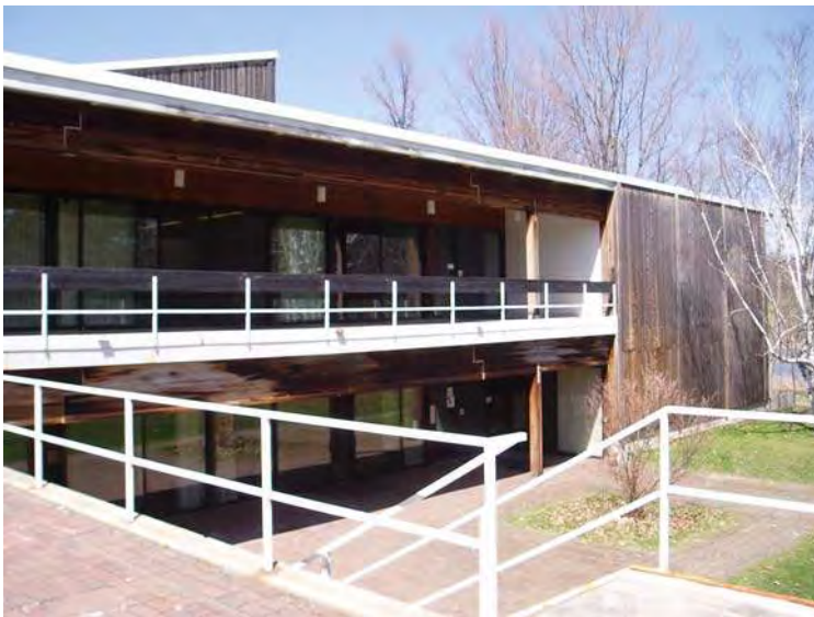
View of east elevation.
