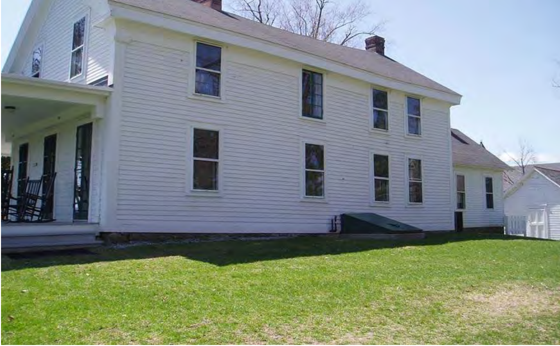
North elevation looking southwest.
