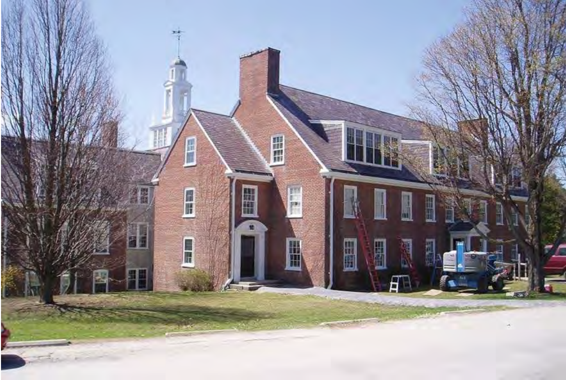
View looking southwest at rear elevation.
