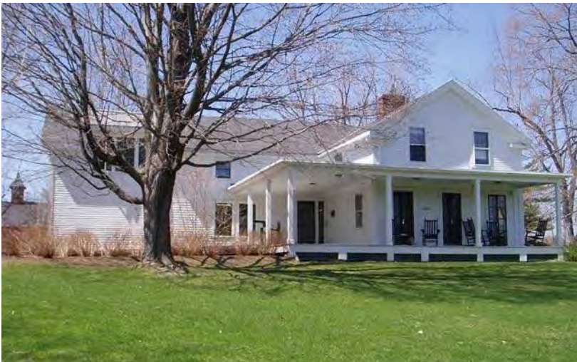
Front elevation looking west.
