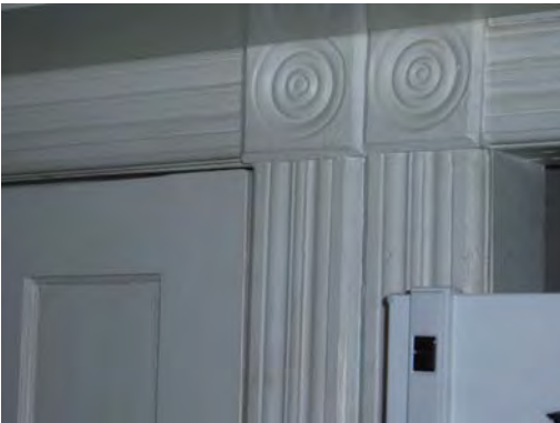
Detail of molded trim with bull's eye corner blocks.
