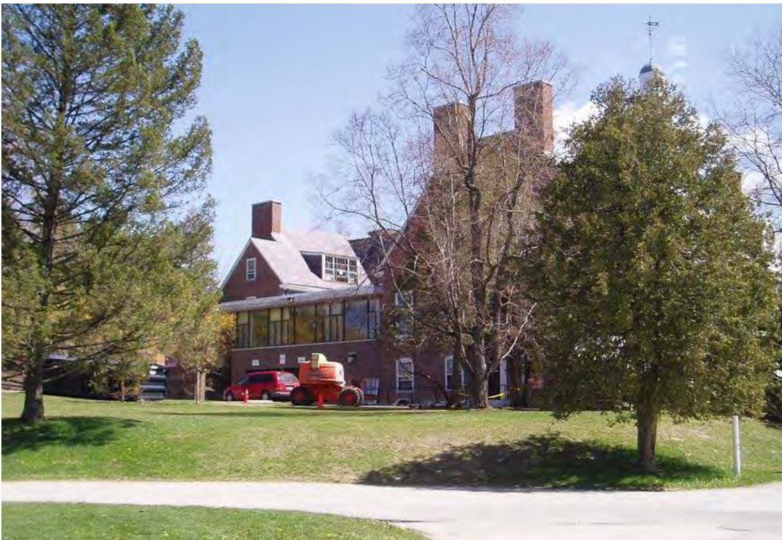
View of west elevation and c. 1965 dining room/ mail room addition.
