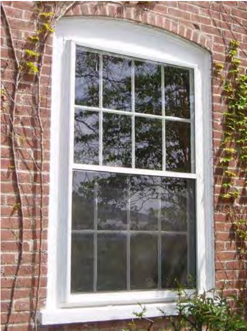
Historic windows: Left photo of eight-over-eight window with wood brick mold, modern storm window. Note grapevine joints in brick masonry. Right photo of original steel window in shed dormer.
