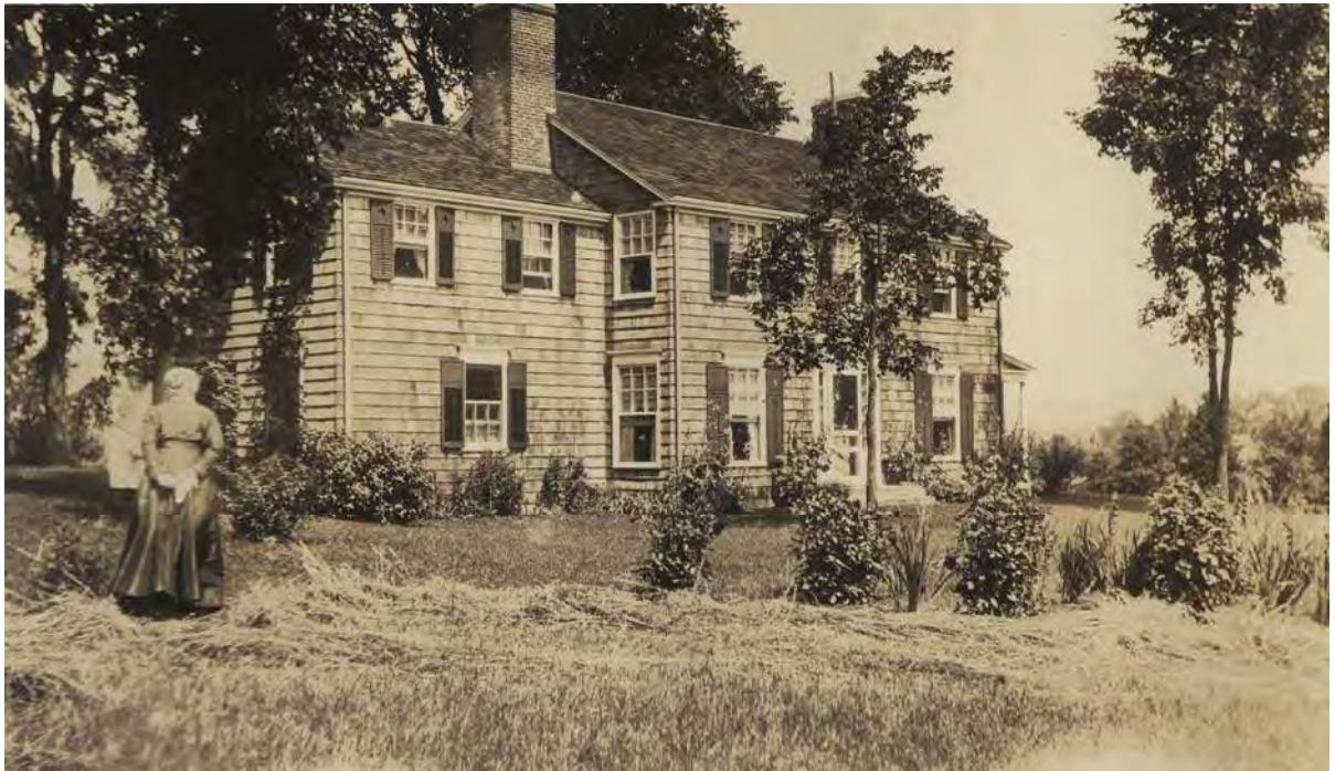
Archival photograph of south elevation with surrounding plantings, and mown field in foreground.
