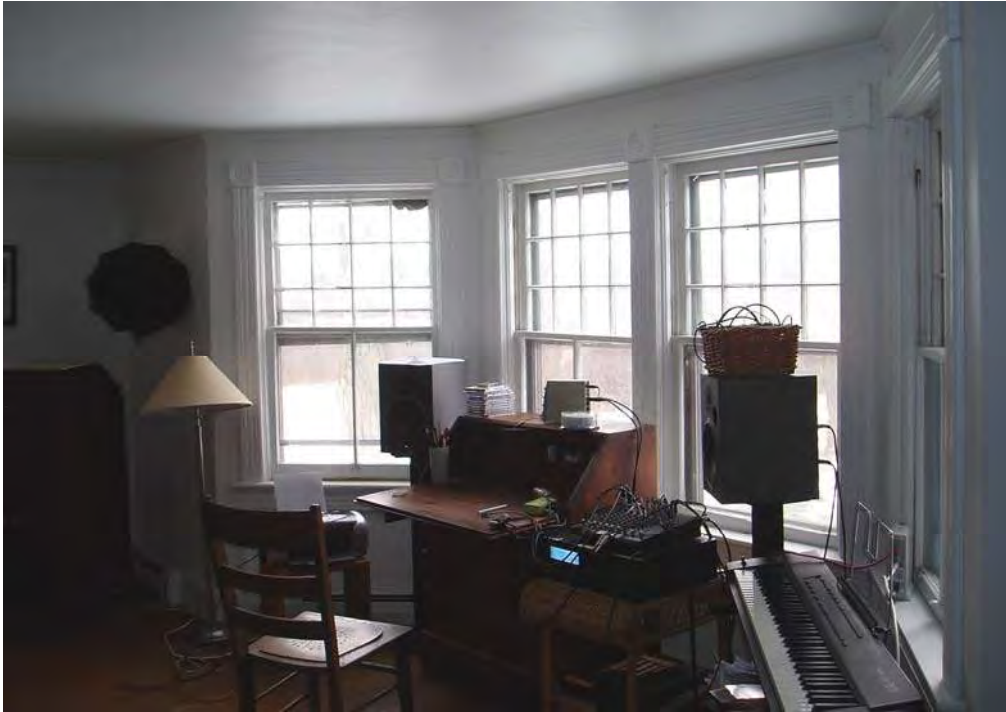
Wing interior, view of bay window.
