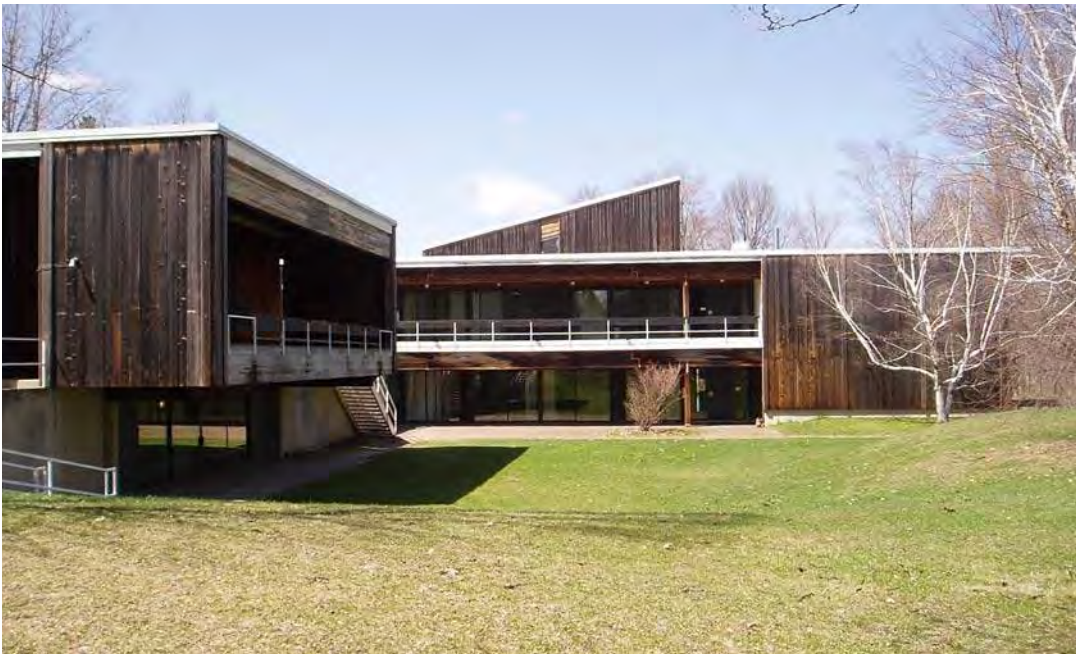
View looking west; Tishman on left, Dickinson Science Building on right.
