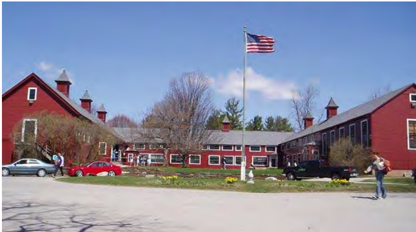
Current view looking north toward west and east wings and center connector.
