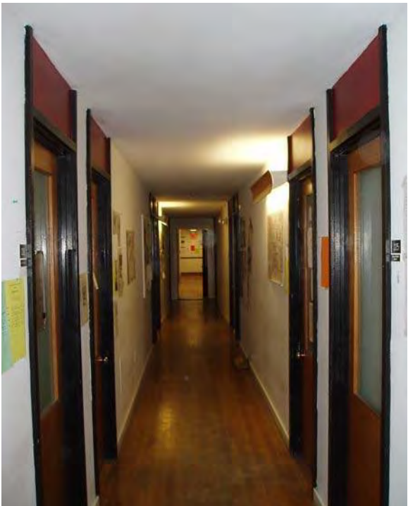
View of east wing north end on second floor.
