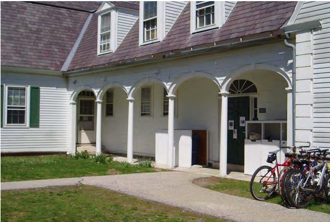
Leigh House (#20) showing the arcaded recessed porch.
