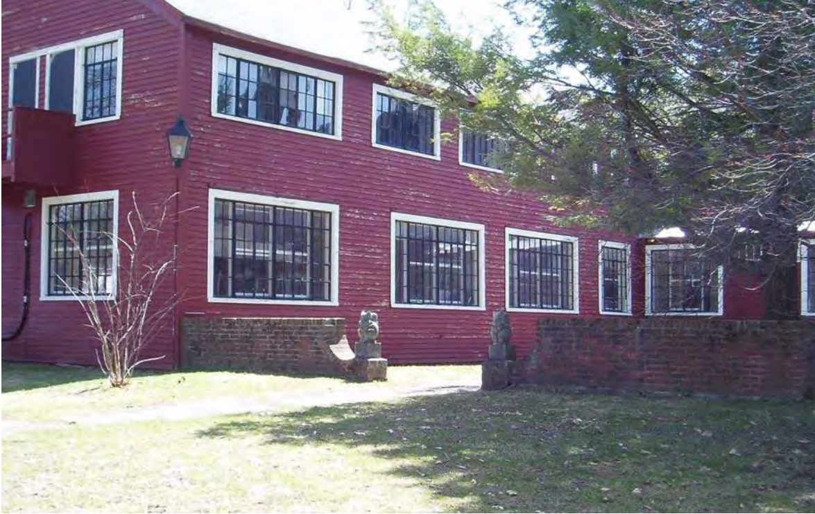
View looking southeast of north end of east wing and brick walled garden area.
