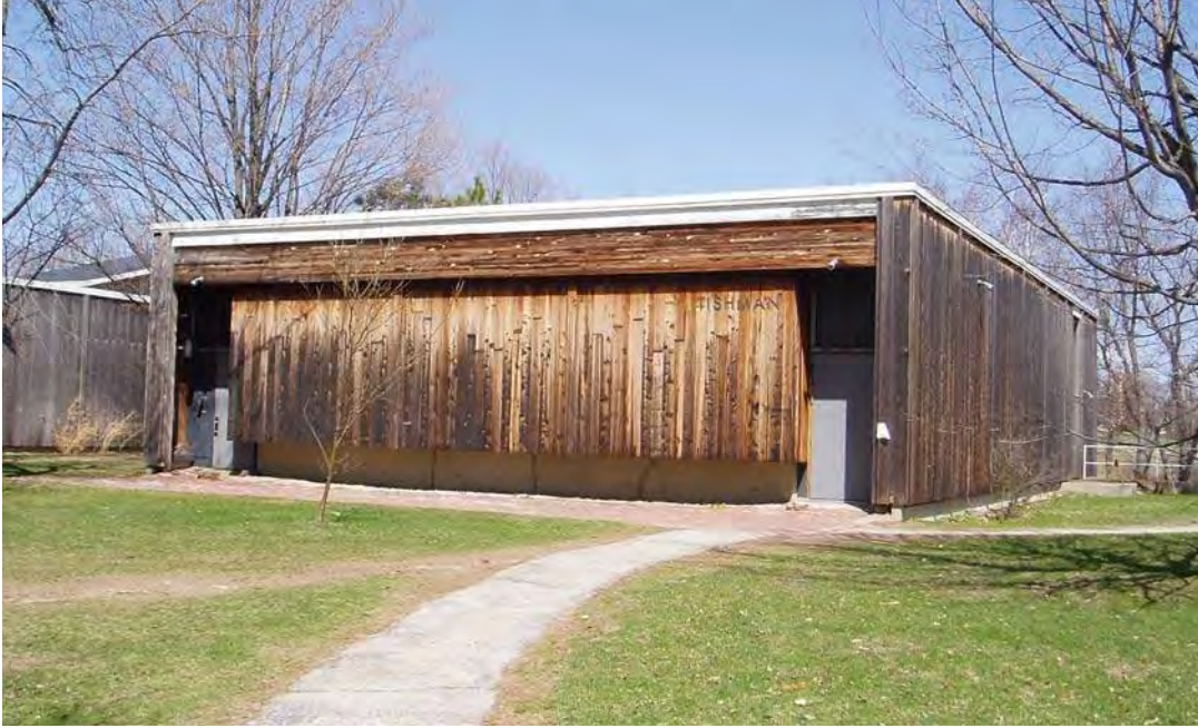
View looking north of front elevation.
