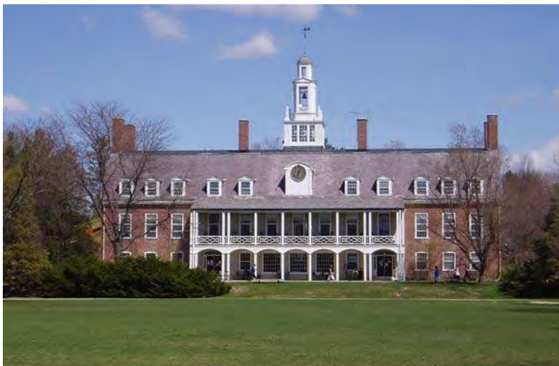
View from the green looking north to front elevation.
