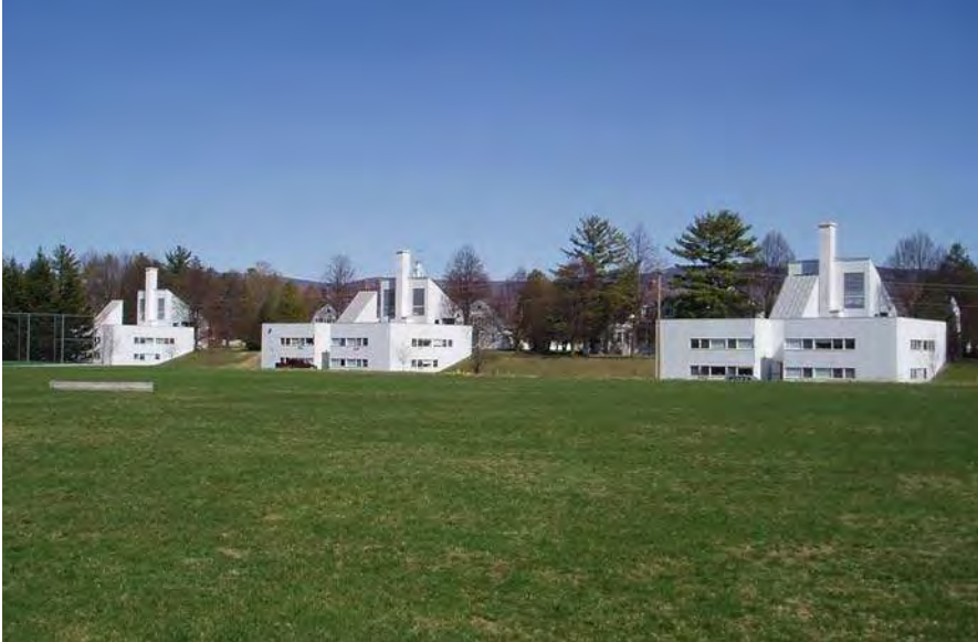
View looking northeast of rear elevations.
