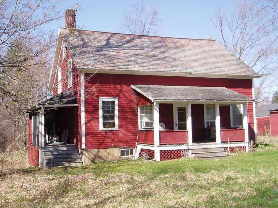
View looking north; walled garden at rear on right.
