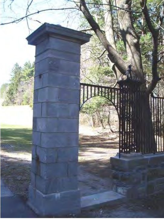
Detail of the limestone post and arched opening for the walking path.
