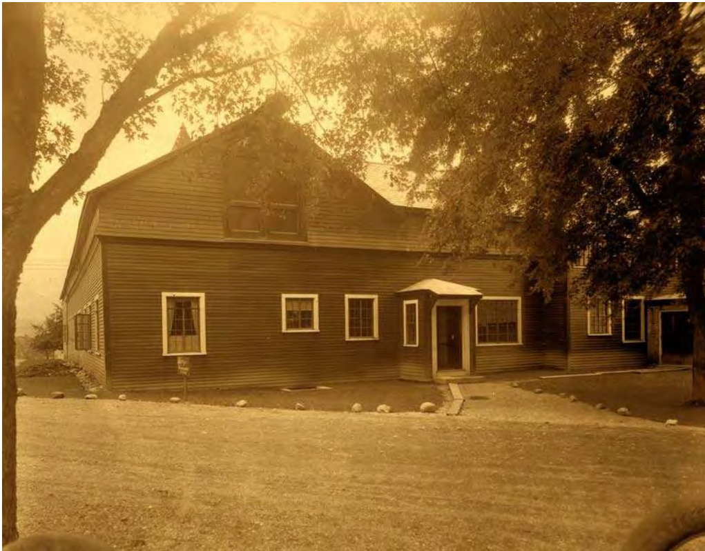
Archive image, Fall 1930 , west wing, west elevation prior to College addition on north end of wing. Note the upper story with intact double hay door in gable and wood shingle siding with a flared beltcourse, a feature that remains today (2007) on the Deane Carriage Barn.
