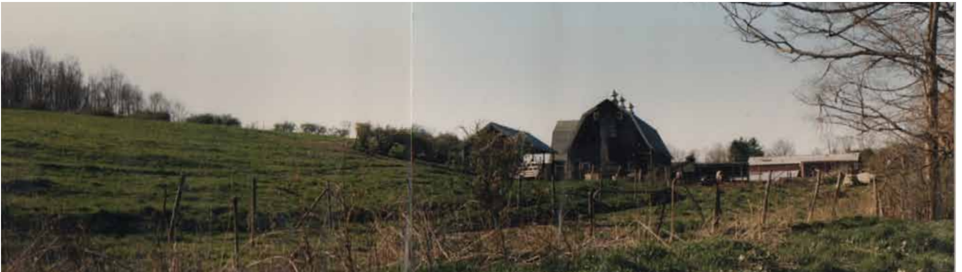
Looking northwest from park street. The milking parlors, manager's house and other support structures.
