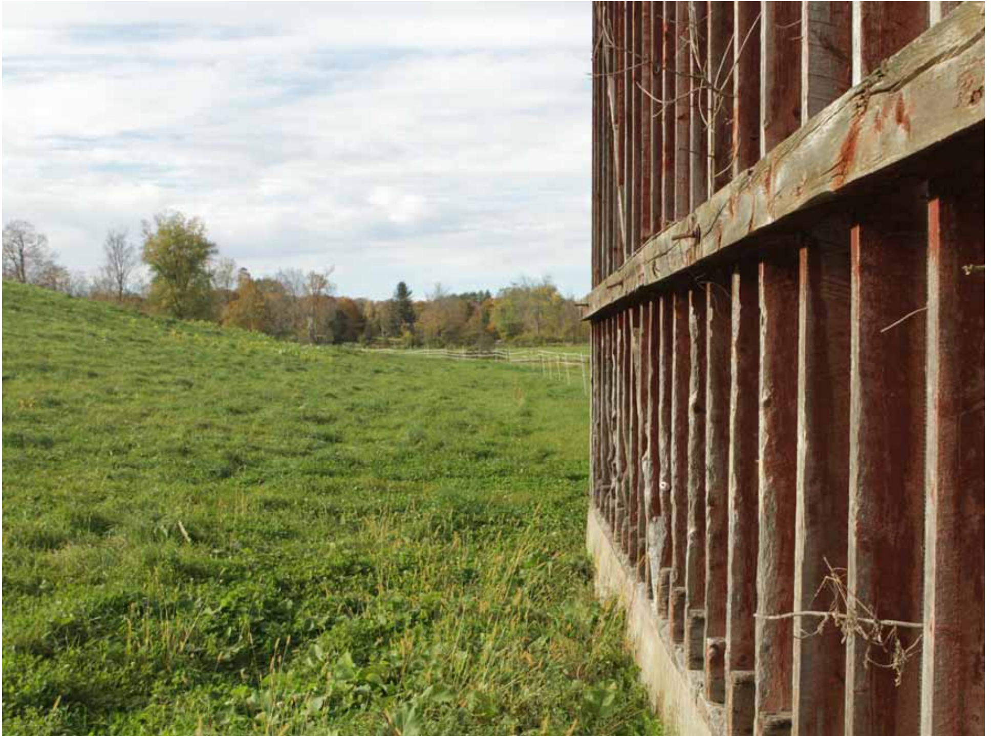
26 View of the hillside and west face of the Corn Crib, 2013.
